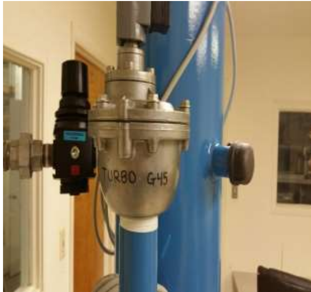
GOYEN PULSE VALVE WITH TURBO G45 REPLACEMENT DIAPHRAGM KIT
