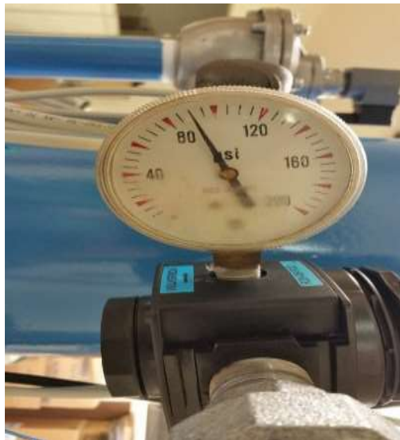
PRESSURE GAUGE ON AIR LINE AT TEST RIG INDICATING 90 PSI
